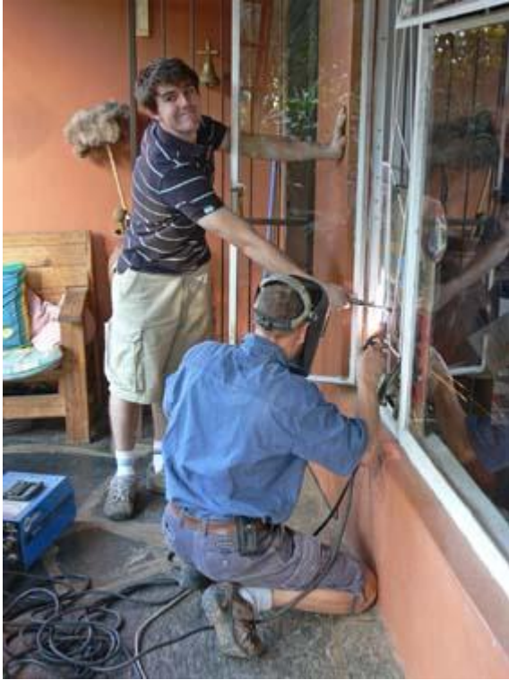
Matthew helping to weld the burglar bars back on.
