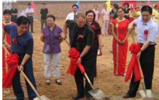
Digging the foundation. Mr LQ Yu, (Luoyang Civil affairs dir.) Robin and Mr Y Lu. (Dir. of CCAA)
